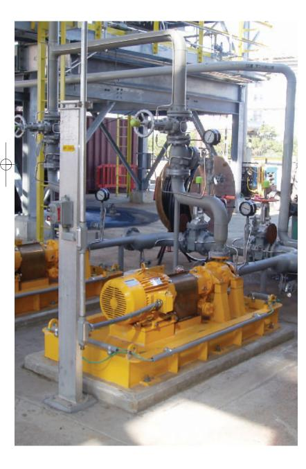
The GSP range comprises of pumps based on the HMD Kontro GS drive, built to API 685 specification, suitable for heavy-duty applications.
