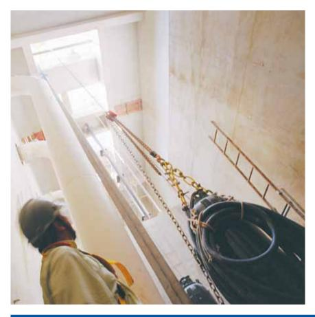
Wastewater treatment plants always need pumps for proper operation. From lifting the sewage up to the plant elevation to pressurizing the effluent against a river at high water, there are many different requirements for wastewater pumps of all sizes.
